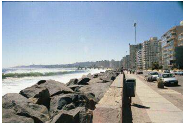
Figure 1 - Condos and Seawall in Valparaiso
